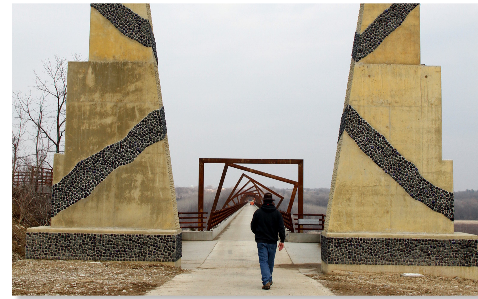
High Trestle Bridge. Source: Mary Swalla Holmes
